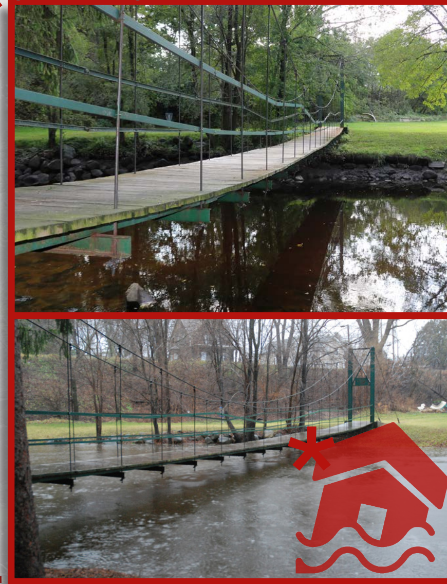
Figure 43, Olen Park Bridge, Michael Walsh
